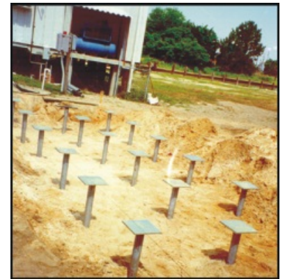
Tank Base Foundation
