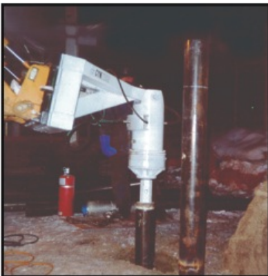
Congested Area Installation
